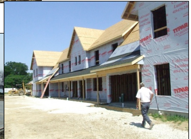
A recent photo of the building. Shingles have almost been completed since this photo, with siding scheduled to start soon.
