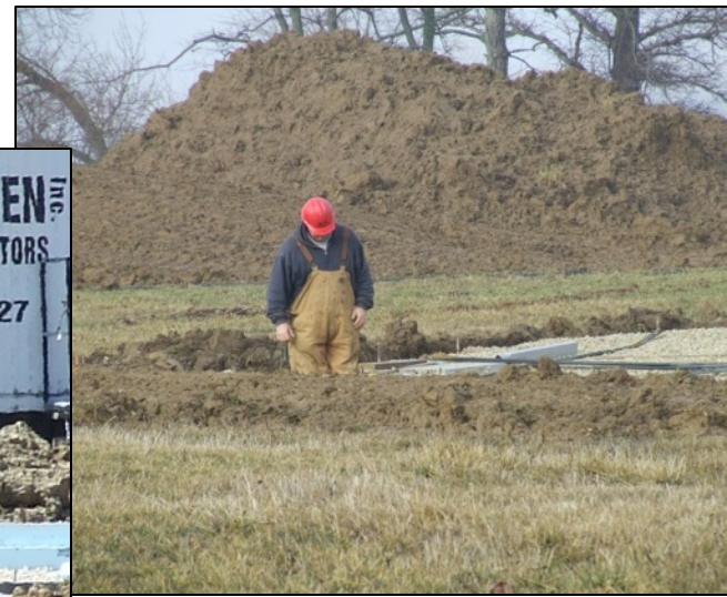
Pouring the building foundation
